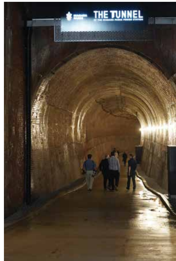
▲ The Tunnel is a pathway 180 feet below ground, inside the former waterway to the Niagara River. Visitors walk the 2,200-foot channel to reach the viewing platform.
